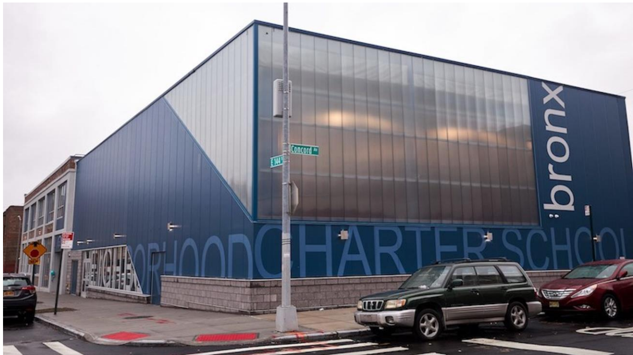
The 58,000-square-foot Neighborhood Charter School in the Bronx borough of New York City, occupies a former warehouse. Photo credit: Transwestern
